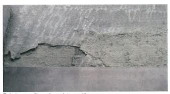
Existing spalling of sandstone sills.
