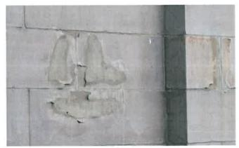
Existing spalling of sandstone blocks.
